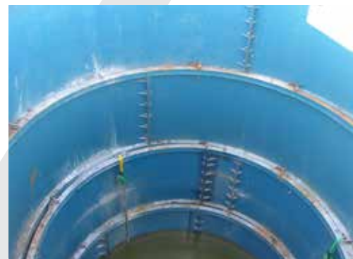
Vertical Shaft Lining
